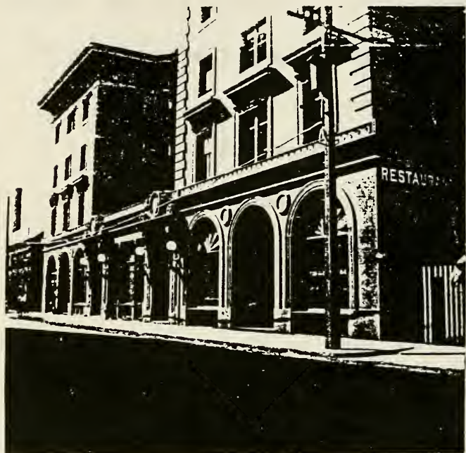
Cambridge Savings Bank Holyoke St. Demolished
